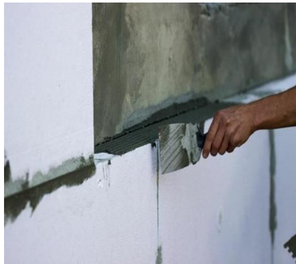
Fig. 9. Apply Grouting
