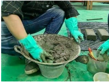
Picture 1. Mixing of Materials
